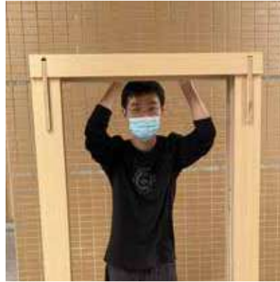
3. Install the top cover on the column to complete the frame assembly
