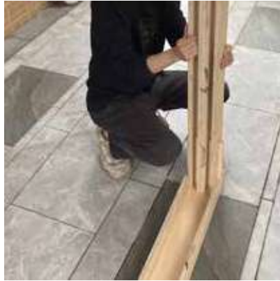
2. Insert the column into the ground slot
