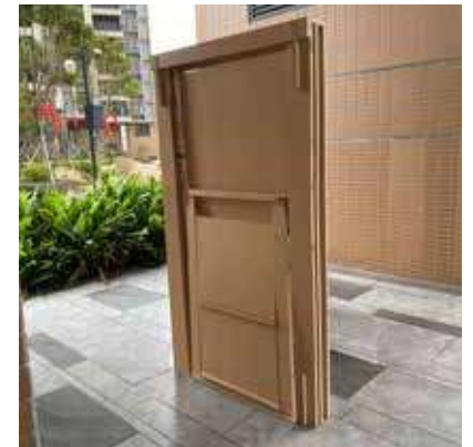
10. CONWALL assembly completed
