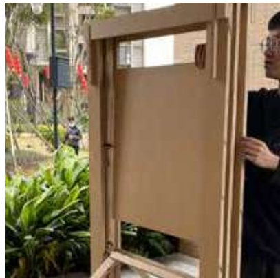
6. Mount the desktop panel to the frame
