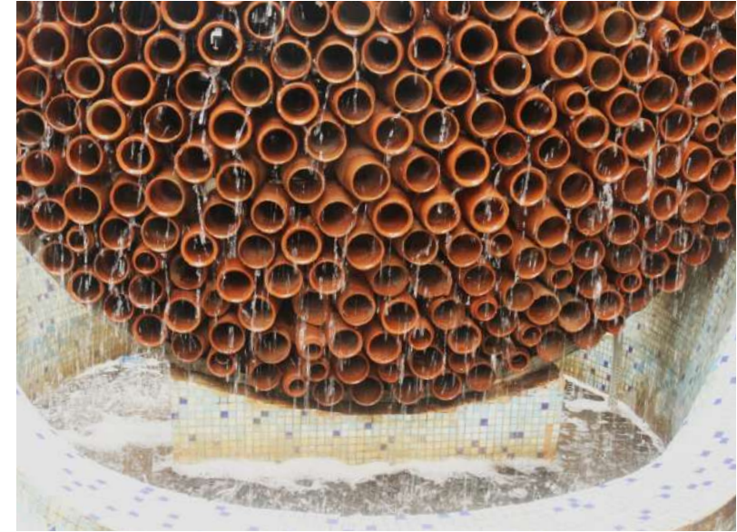
Terracotta structures that offer a natural way to cool air, designed by Ant-Studio.
